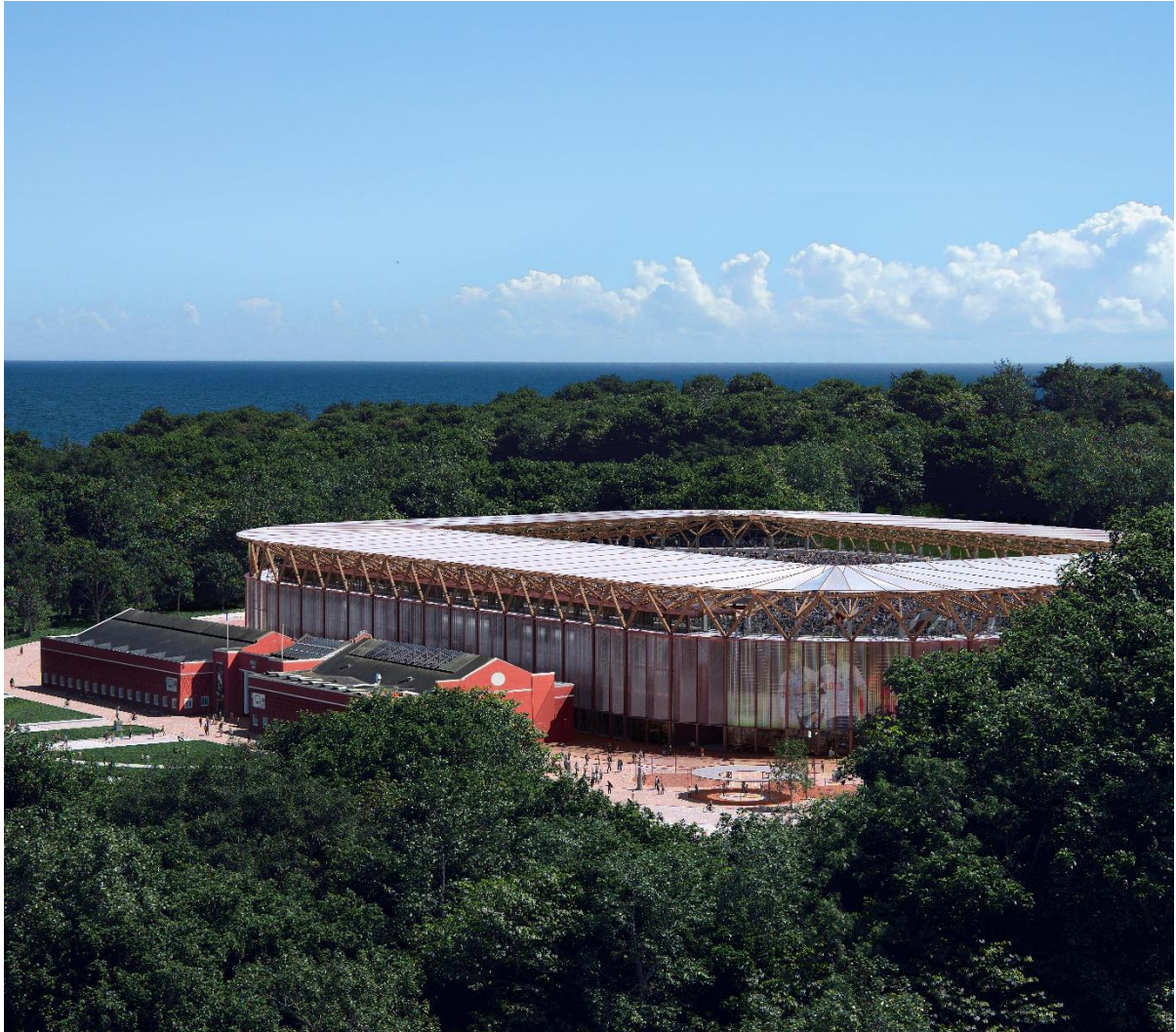
New Aarhus Stadium_“Under the tree tops”
