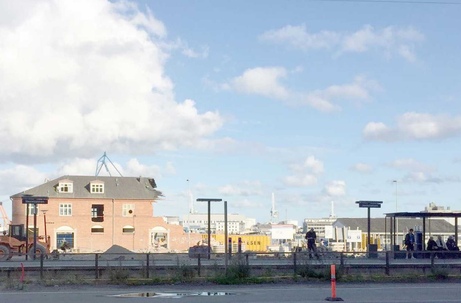
Pakhus 27 nedbrydes, september 2015.
