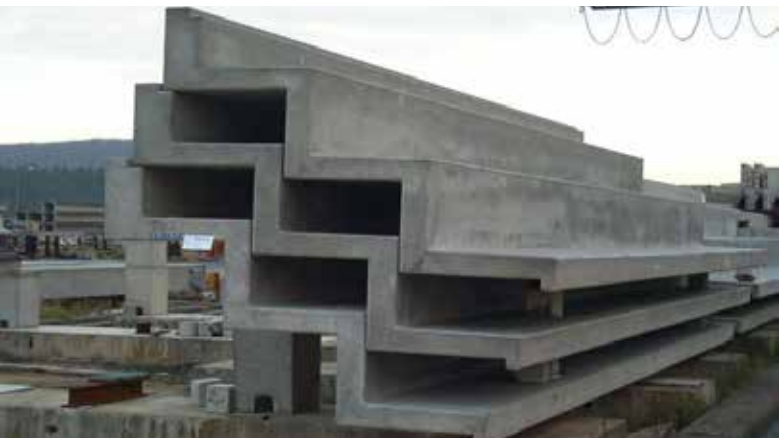
New precast concrete steps for lower rows of the stadium bowl and for main stand terracing
