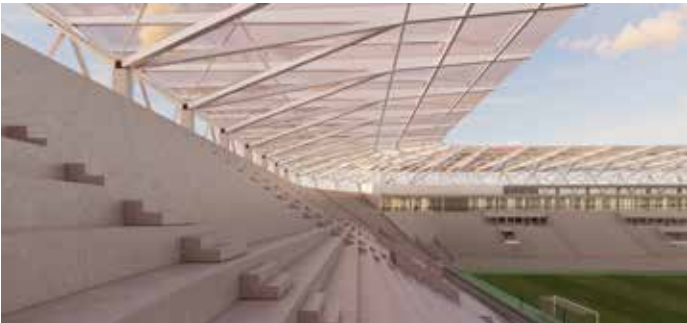
PHASE 2 - PRELIMINARY PROPOSAL Steel truss – PVC textile & ETFE foil
